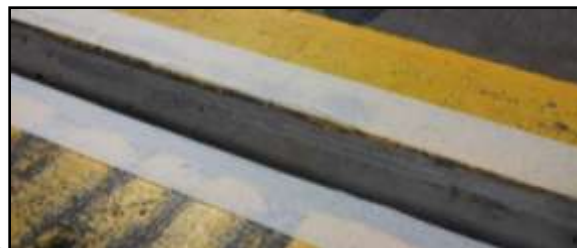
2. Expansion joint masked and cleaned
