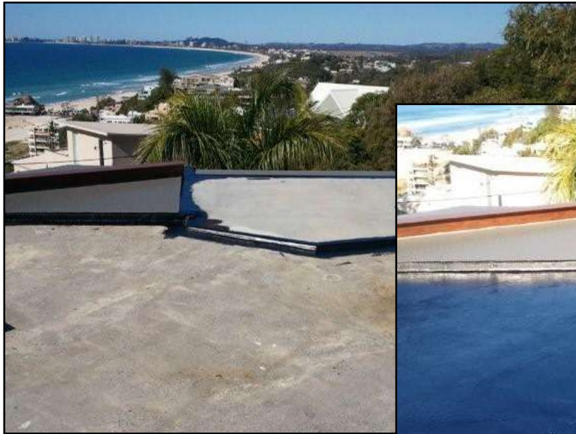
1. RTT Sealant applied to joints and corners
