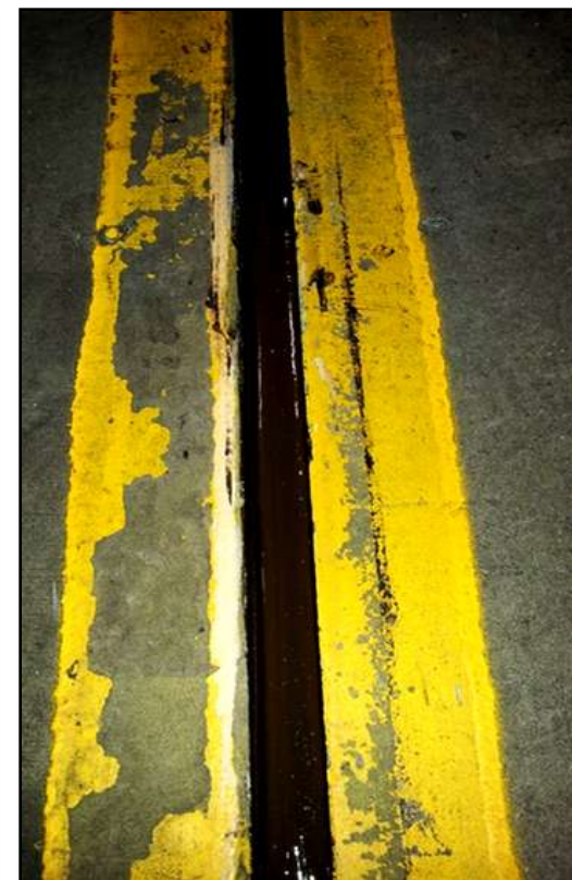
RTT Sealant poured in to seal and close joint
