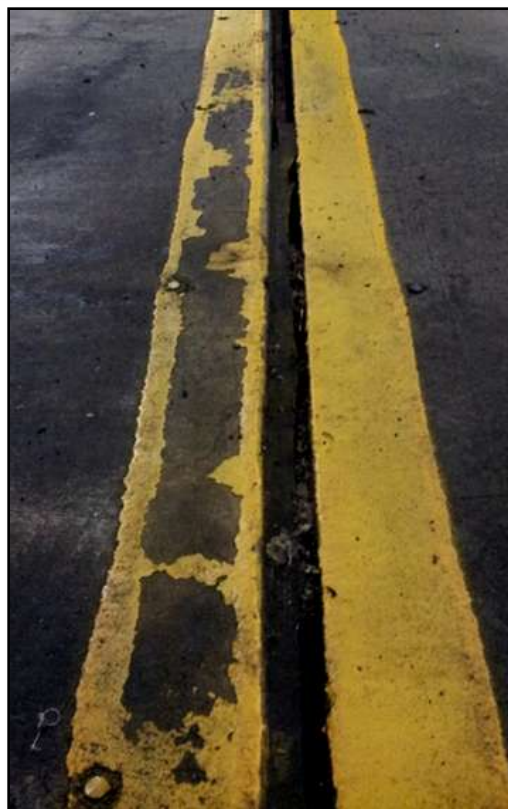
Existing joint sealant to be removed
