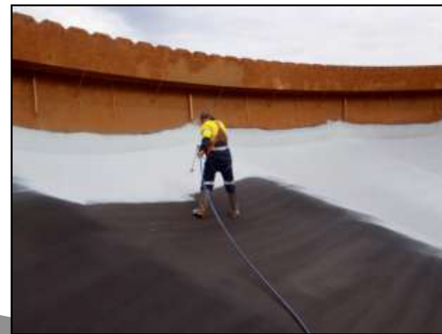
RTT Sealant being spray applied
