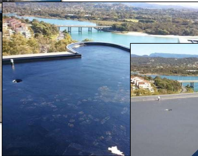
2. RTT Sealant applied to entire area
