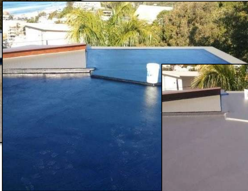
2. RTT Sealant applied to entire area
