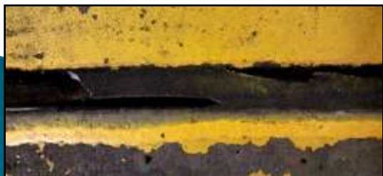
1. Existing seal to be removed
