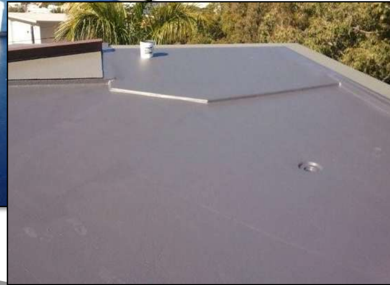
3. Coloured top coat applied to RTT Sealant
