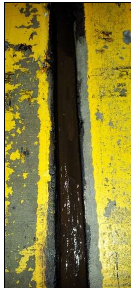
3. RTT Sealant poured into empty joint
