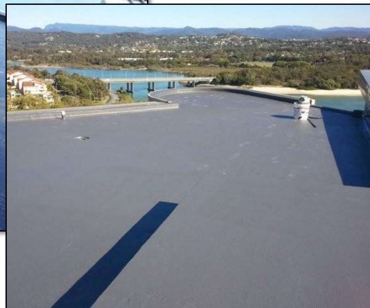
3. Coloured top coat applied to RTT Sealant
